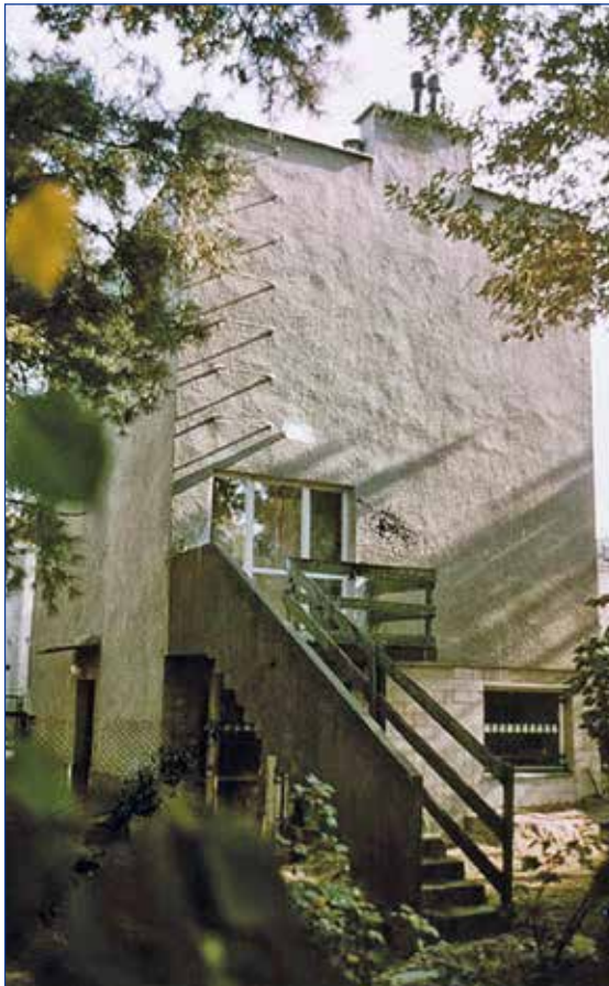
The Nowicki family house in Warsaw – present day. First design by Maciej Nowicki from the beginning of the 1930s. The house was rebuilt after 1945, and its original features were lost in the process. (photo: Tadeusz Barucki)
