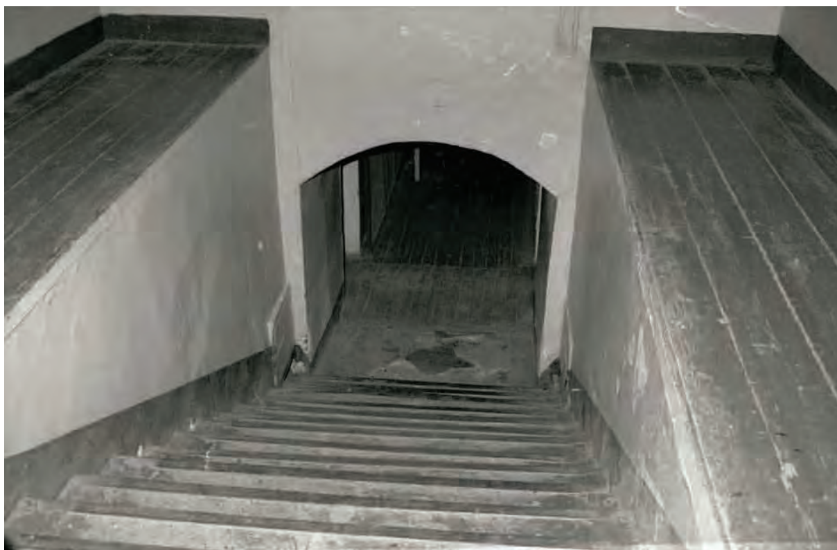
Stairs leading to the basement. (Photo Aleksander Załęski)
